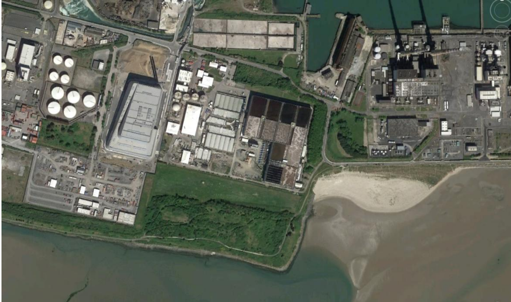
Aerial view over Ringsend site.
